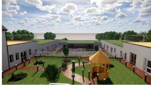
View from First Floor Bedroom
